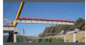
Bridge beam and edge protection lifted into position as a single unit.
